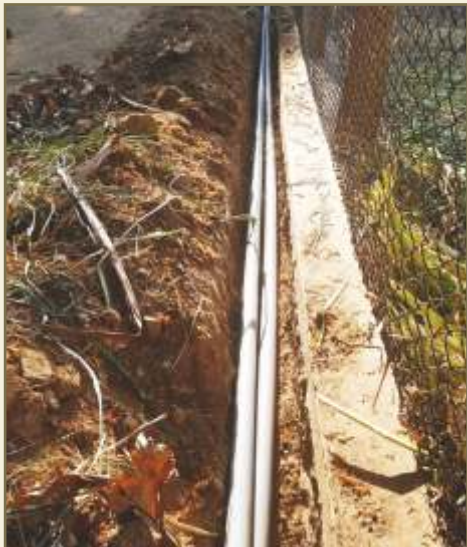
B 6. Installation of Jet Sprinkler at Deer Enclosure
