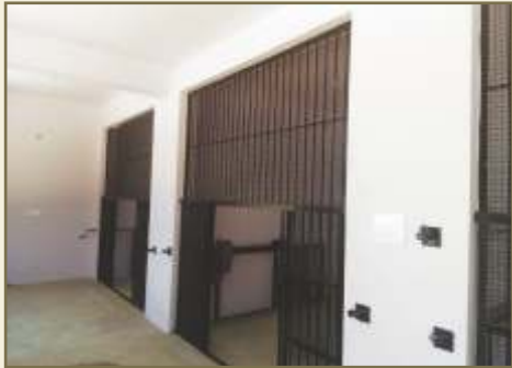
B 5. Construction of Jaguar Enclosure at Zoo
