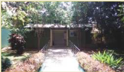
Renovation of Toilets
