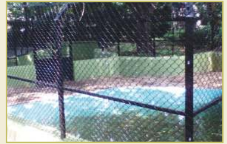
Renovation of salt water crocodile enclosure
