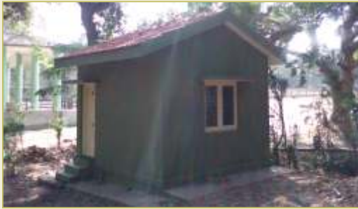
Construction of keepers room near African Elephant enclosure
