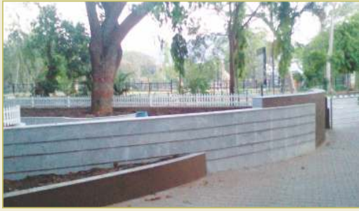
Food court renovation at Amphitheatre
