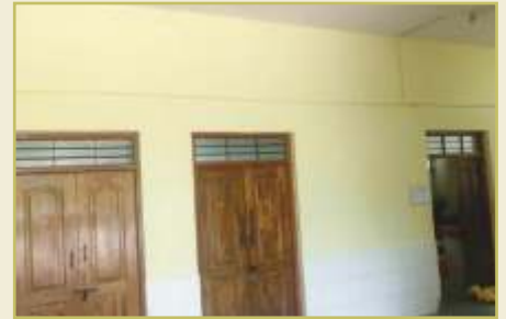
Painting Work at Store
