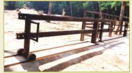
construction of iron railings at Indian Elephant Enclosure .
