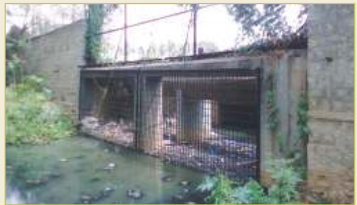
Providing Gates to storm water drain
