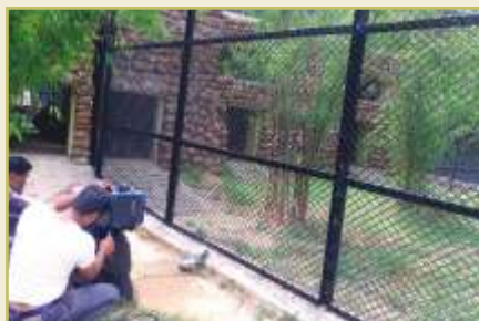
Lion Enclosure Double Mesh : We have two lion exhibit areas, usually the lion tends to fight with other lion which are another side of the exhibit areas. We have recorded couple of issues with minor injuries so double layer mesh was laid all along the exhibit & day kraal areas where the lions are come in contact with each other.
