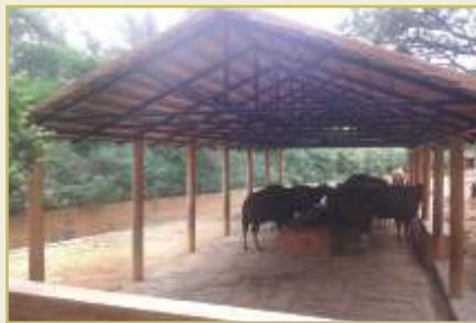
Guar Shelter : Shelter with Mangalore tiles was constructed at pen 1 Guar enclosure to provide protection from rain and hot sunny weather.
