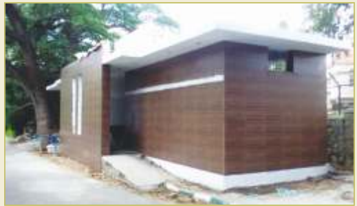
Construction of rest room at Giraffe Enclosure
