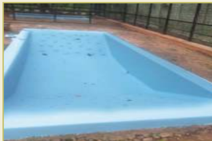
Tiger enclosure: Water ponds are constructed at Tiger Day kraal areas to provide them a natural environment and as part of enrichment.
