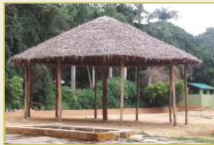
Rhino Enclosure Pergola: Thatch roof pergola was constructed inside the Indian Rhino enclosure to provide shelter from sun and rain.
