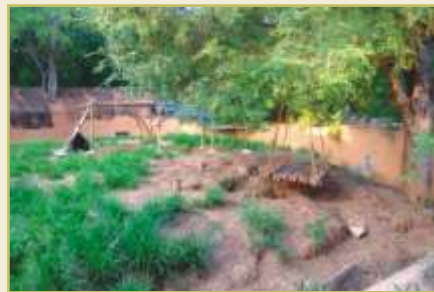
Enrichment Work at Bear Enclosure: Roller drums, See-saw, Swing & Hammocks were installed at two sloth bear enclosures. The Bears loves to use all these enrichment articles & this attracts public in larger way.
