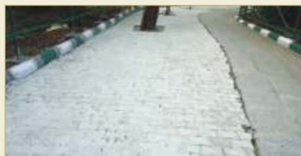
Widening of the path
