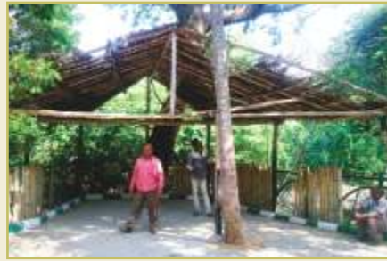
Visitors shelters made out of thatched roofs using coconut palms
