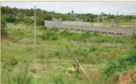
Strom water inlet Koorgahally
