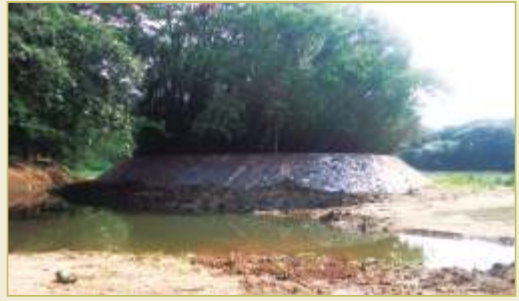
Karanji island revetment
