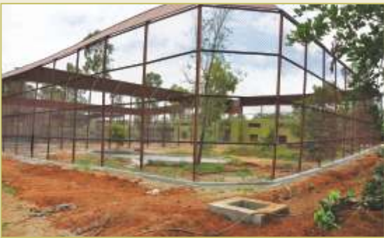
construction of day kraal
