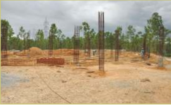
Hospital under construction, Koorgahally
