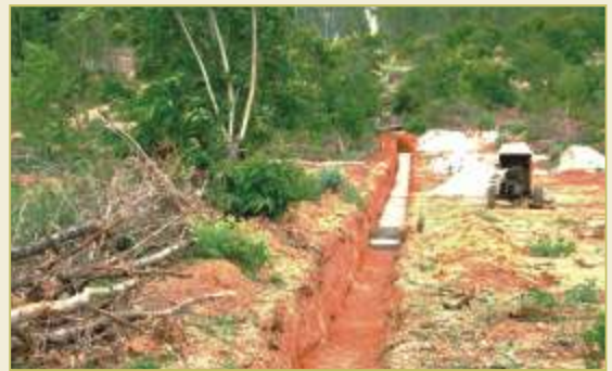
Gaur enclosure under construction
